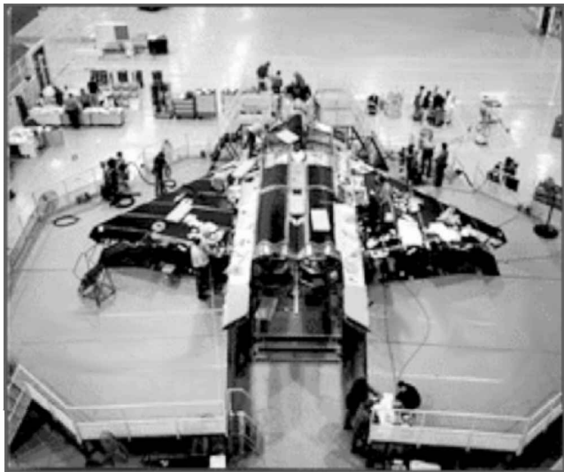
Fig. 8 Assembly of F-22 composite wings.
